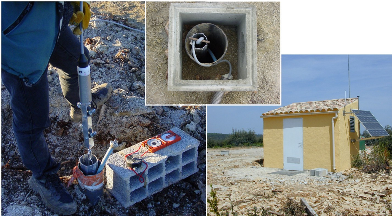
Geosig triaxial sensor during installation
